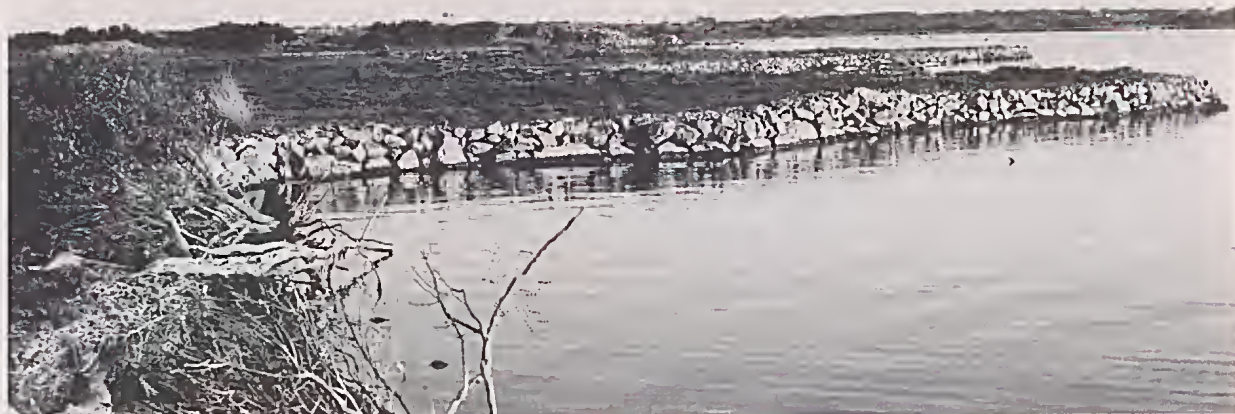
Fig. 6—Rapid shoreline erosion on the Mitchell delta has been halted by the dumping of granite and sandstone boulders to form a protective shoreline wall. Photo: Eric C. F. Bird.
